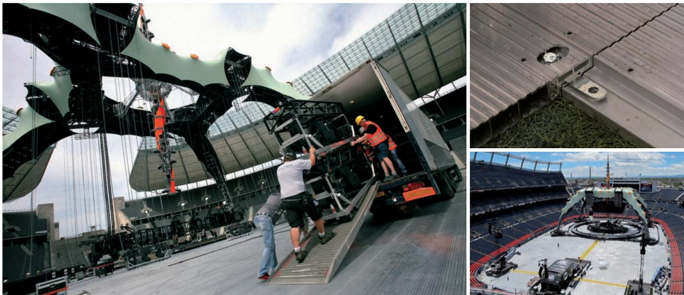
U2's 'Claw' support rig sits on eps's Arena Panels, which are secured with counter-sunk bolts (top right) to create a stable base
